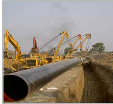
Crude Transmission facility 24" Dia - Yukse Co.Ltd Munifa to Razal Zour 89 KM
